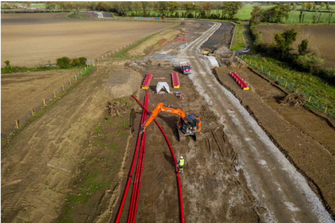
Figure 5.6: Typical underground cable construction in agricultural lands
