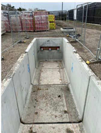
Figure 5.8: Pre-cast Joint Bay prior to Cable Installation
